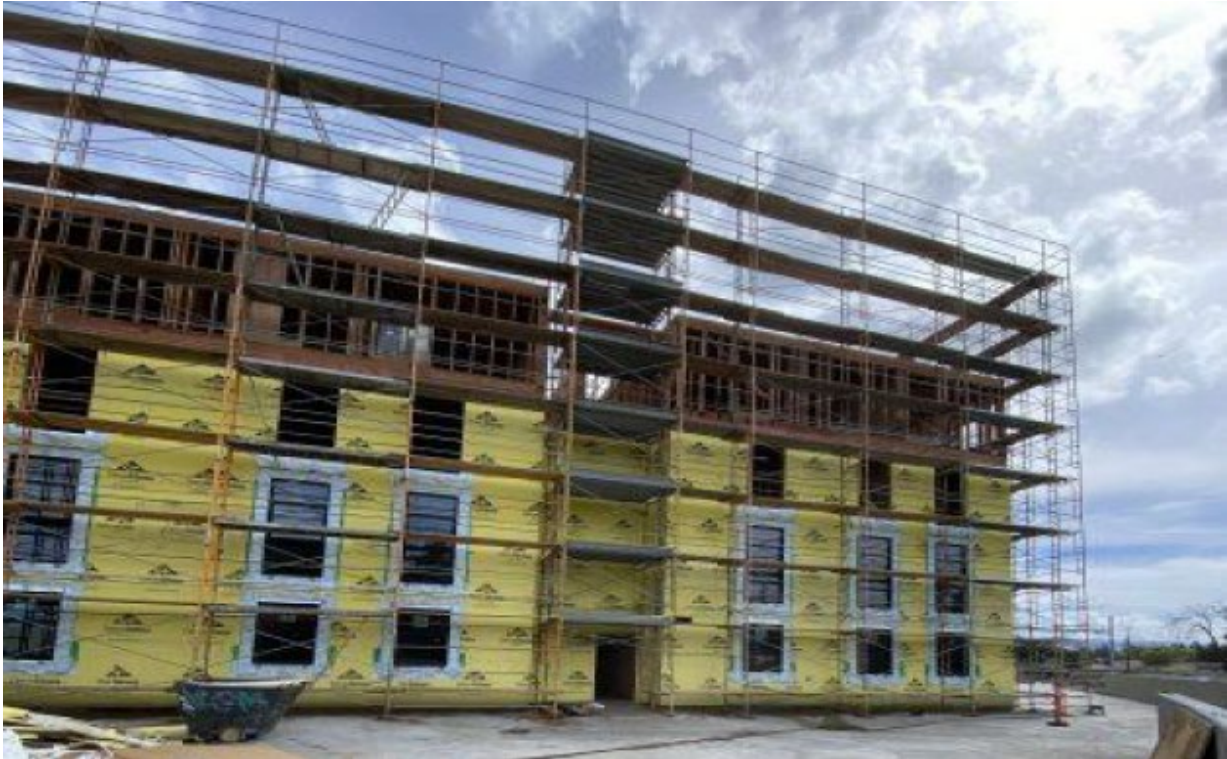
Figure 3 – Window installation progress at the southern building, March 2024.
