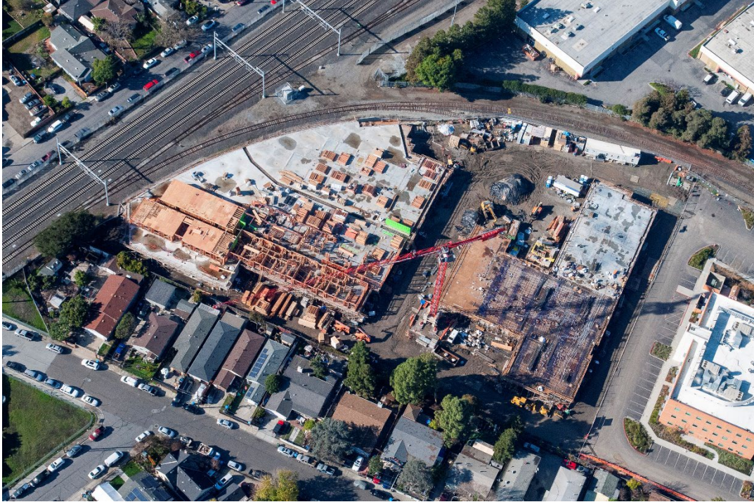
Figure 1 – Aerial view of construction progress at the beginning of January 2024
