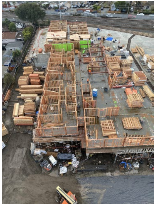
Figure 3 – Framed walls for southern building
