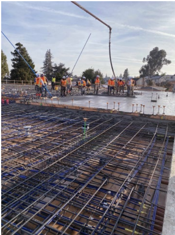
Figure 2 – Installed structural supports (near) and completed section of concrete pour (far)
